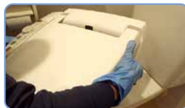
▶ 温水洗浄便座の取付け
